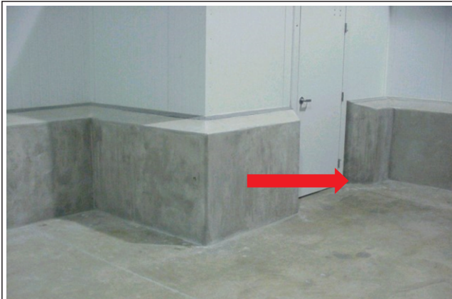
Figure 13: Concrete curbs of essential heights
