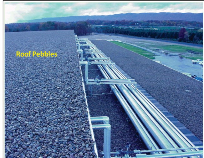
Figure 15: Stone pebbles on the roof absorb and reflect the heat
